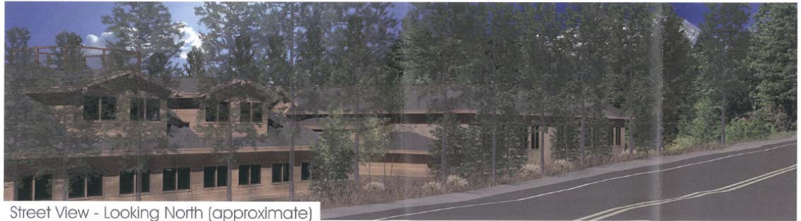
Street View - Looking North (approximate)
